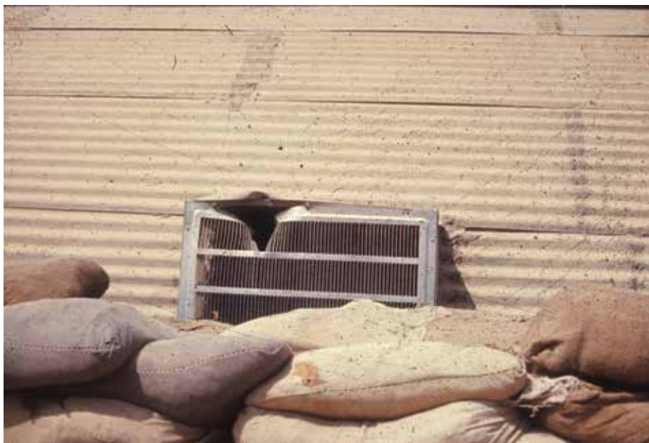
Figure 3-18. Quonset-hut hospital wards at Cu Chi, with sandbag walls against shellfire. Reproduced with permission from: Slide VAS032312, Ivan Dalton Collection, The Vietnam Center and Archive, Texas Tech University.
