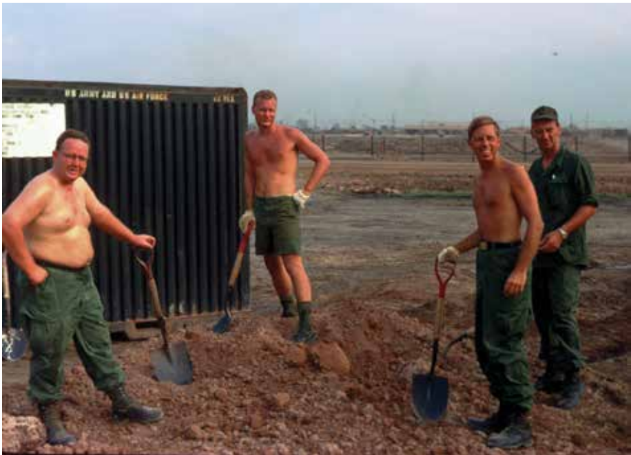
Figure 3-17. Officers excavating for a bunker. Photograph courtesy of Howard Hirsch.
